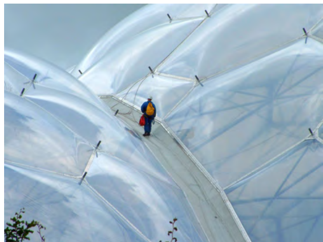
Grimshaw Architects – Eden Project, Cornwall, United Kingdom, 2001 Sources: www.grimshaw-architects.com
